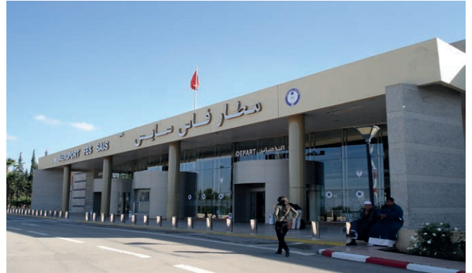
FÈS-SAÏSS AIRPORT - MOROCCO
